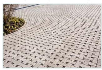
Figure 57: Example of a permeable paving that could be used for driveways.
