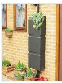
**Figure 59:** Example of a gravity-fed rainwater system for flushing a downstairs toilet or for irrigation.
